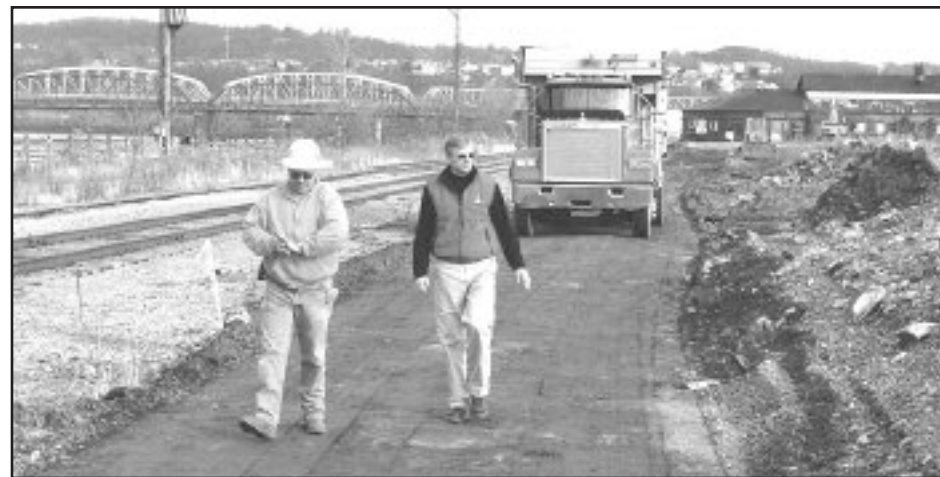
Work begins in McKeesport on closing "the gaps in the GAP."
